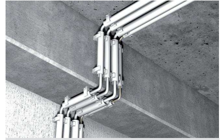
Fixing plastic insulating conduits
